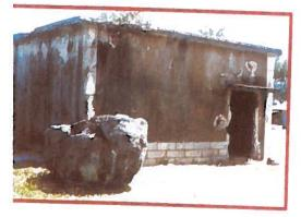
The building is a good extant example of Japanese non-military architecture. The outside of the building was roughed cement-rendered. A bottom section within the exterior walls shows a wainscot, offset by a recess from the roughed cement render. The wainscot is comprised of smoothed render, ruled off in a fashion so as to imitate three layers of masonry. The eaves of the flat-roofed building are protruding, with a cantilevered canopy over the northwestern entrance providing protection from rain.
